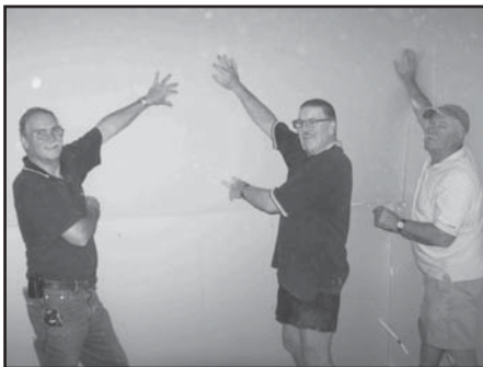
Bendigo Team fitting plaster sheets at Ali Curung
